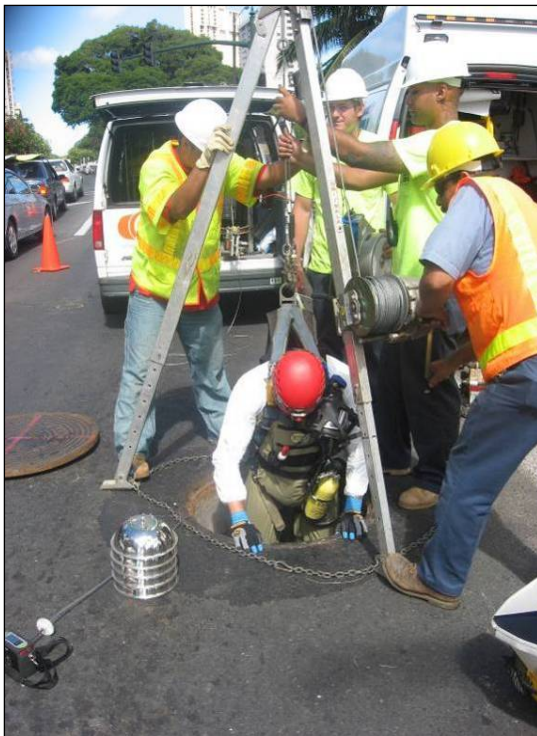
Photo 1. Confined Space Entry
