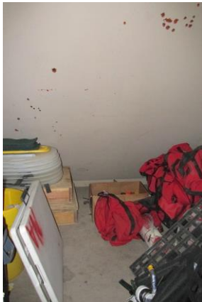
Photograph 4. View of the deflection wall in the former firing range area.
