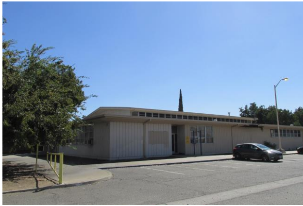
Photograph 2. View of one of the onsite structures, facing southeast.
