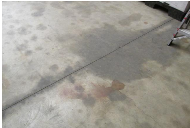
Photograph 5. View of the stained flooring in the former firing range area.
