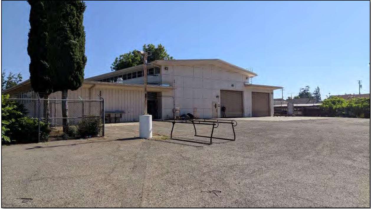
View of the rear elevation of the building located on the site, as seen from the yard space
