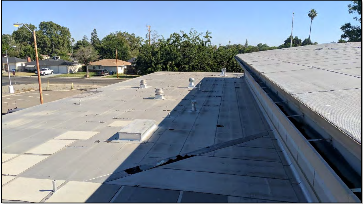
View of the roof deck of the building located on the subject property (typical)
