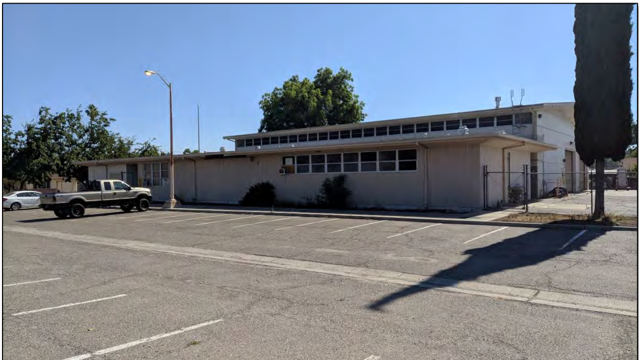
View of the west side elevation of the building located on the site, as seen from the parking lot
