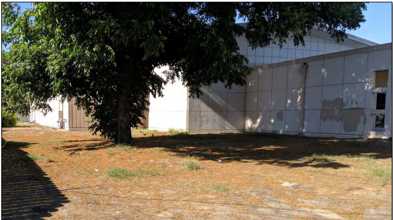
View of the east side elevation of the building located on the subject property, as seen from Flower Street
