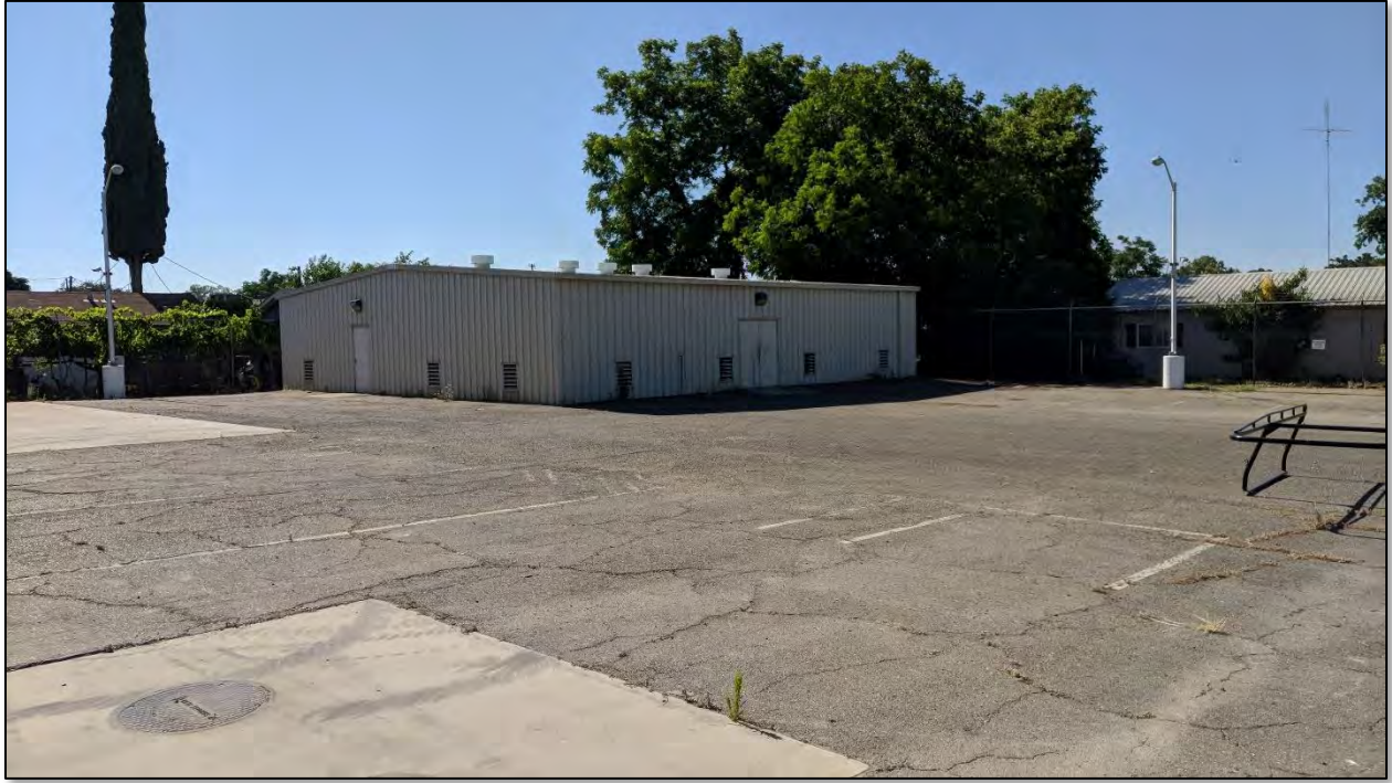
View of the metal utility building located on the subject property, as seen from the yard space
