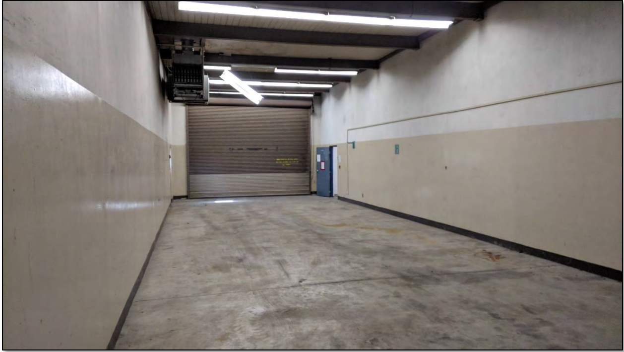
View of the interior "Rifle Range" area of the building located on the subject property
