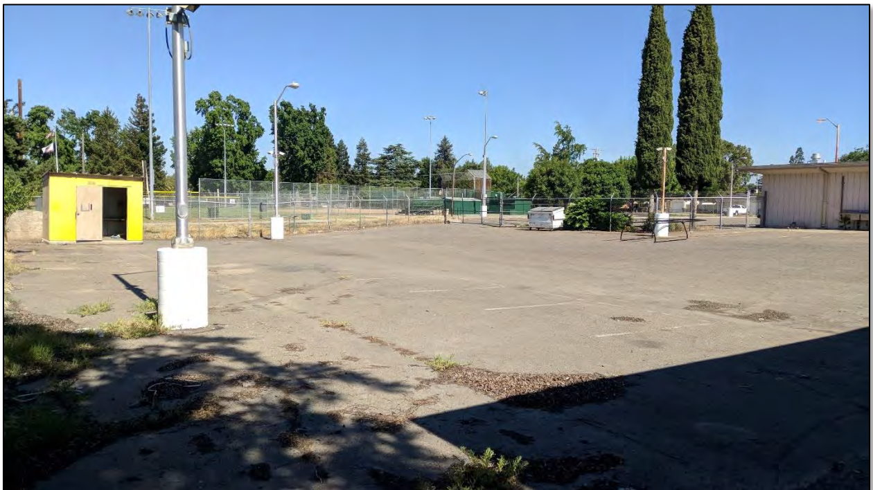
View of the secured yard space, as seen from near the metal utility building
