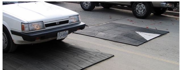
Temporary Speed Cushion
