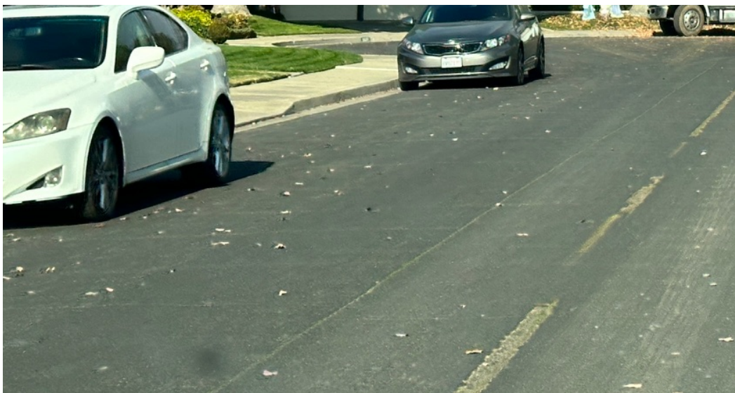
Photo 1: Section 1 Moderate Longitudinal Cracking
