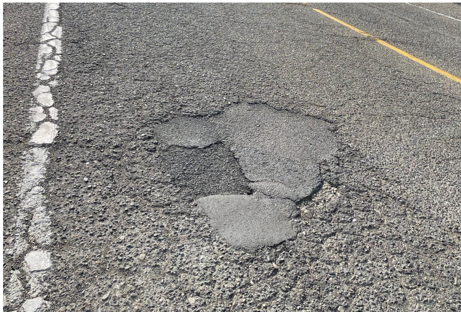
Photo 2: Section 2 Raveling, Alligator Cracks and Failed Patching
